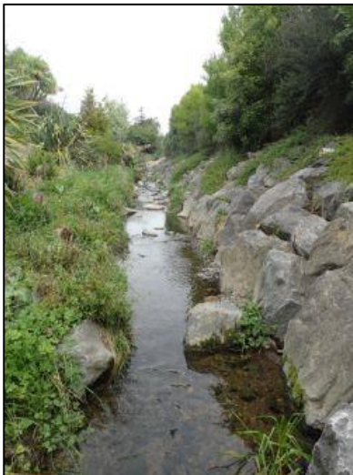
Figure 5. Rock armouring creating pools
