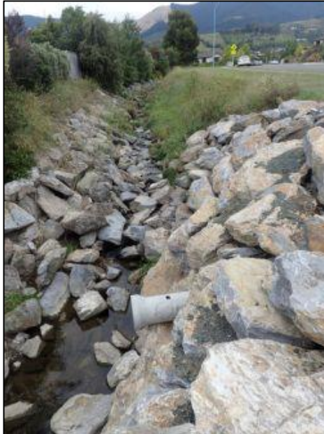
Figure 3. Upstream Kareti Drive Bridge
