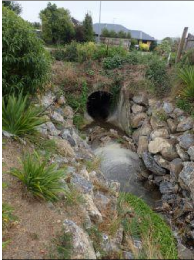
Figure 16. Hill Street culvert
