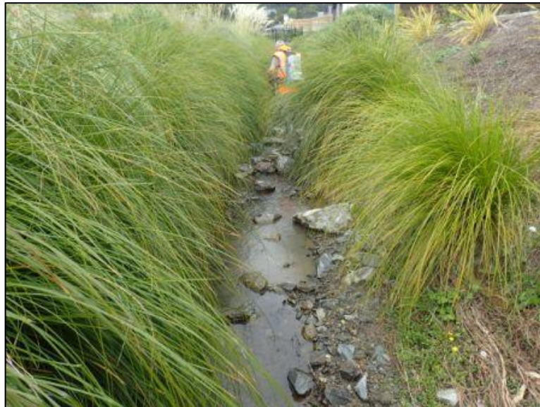
Figure 11. Upstream Hill street culvert
