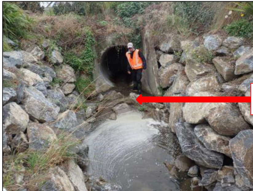
Figure 12. Uplifted filter cloth backing up water
