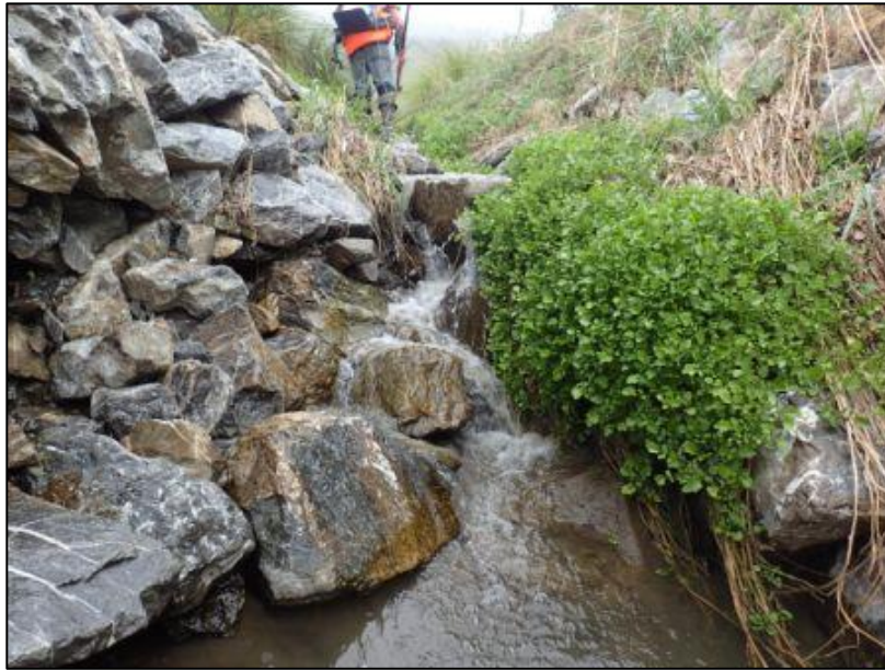
Figure 14. Rock armouring causing a gradient drop in the stream
