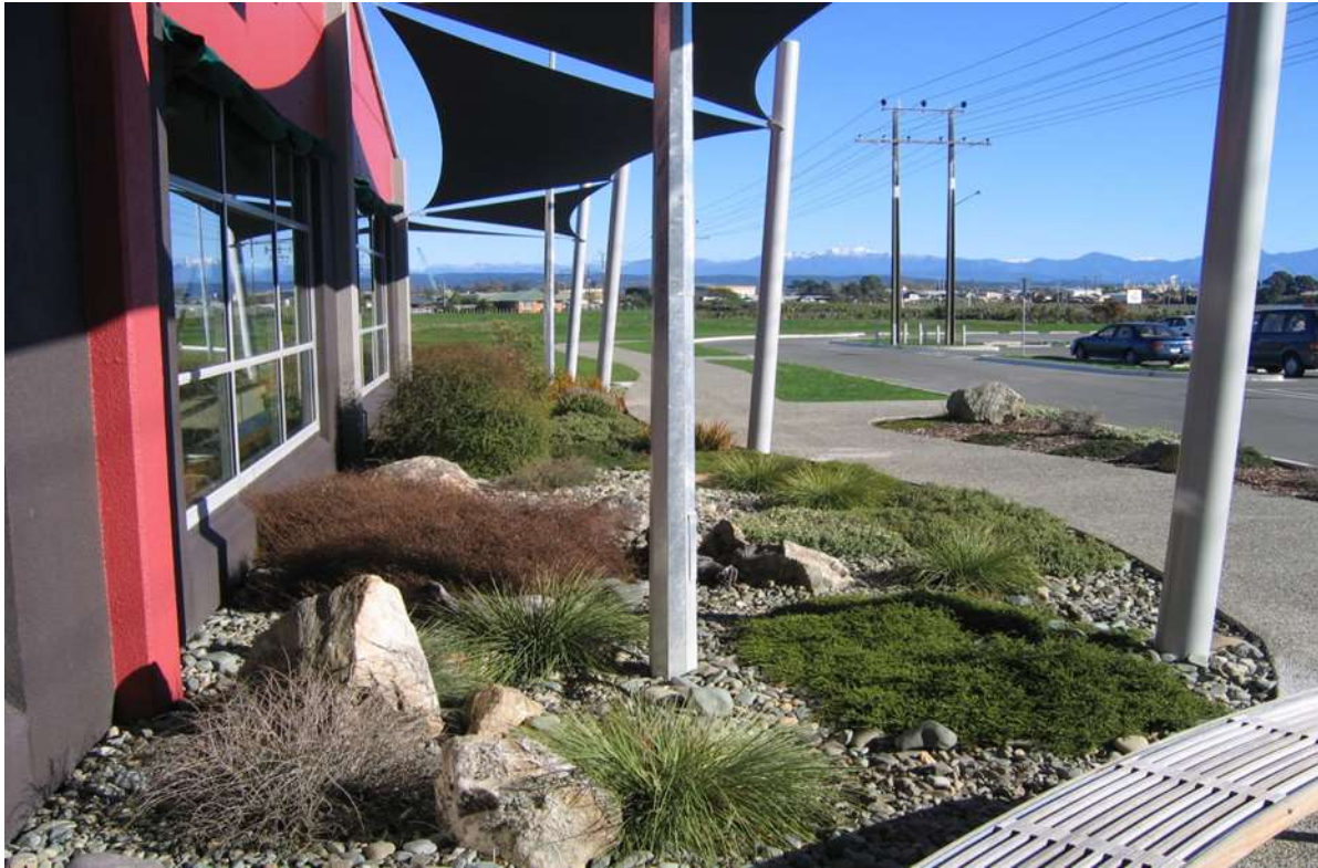
Figure 1: Richmond Aquatic Centre frontage.
