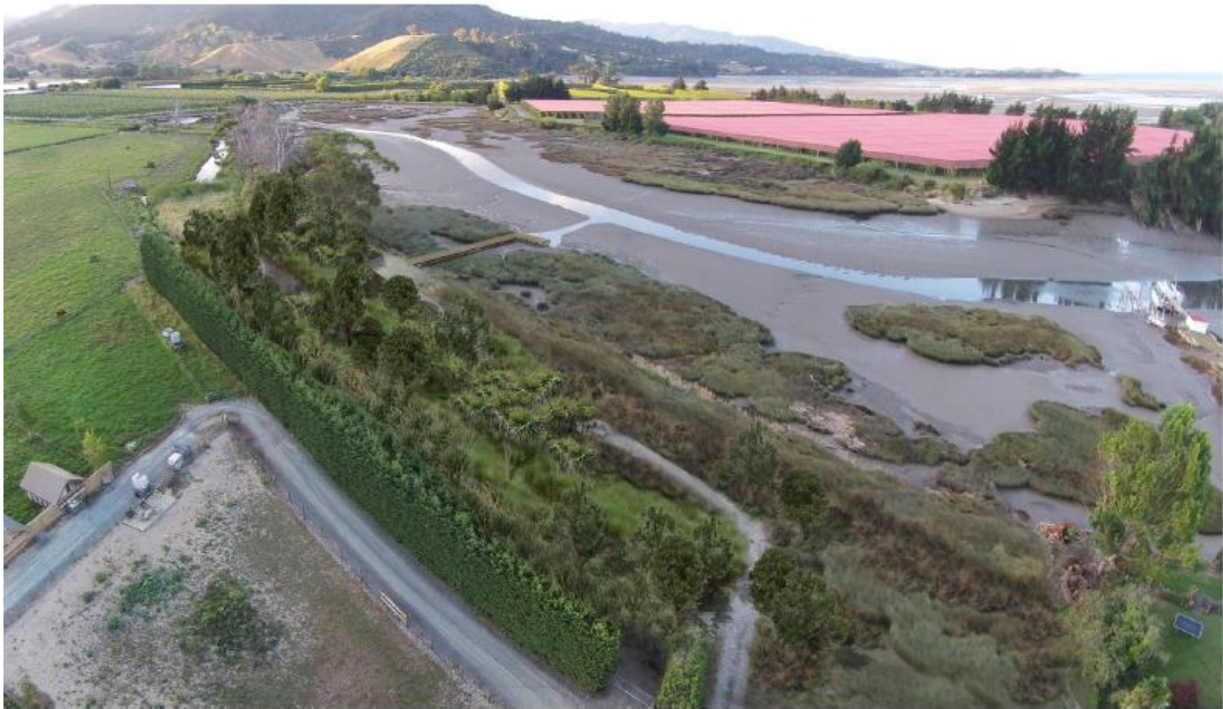
Figure 7: Graphical representation showing the location of the proposed jetty and access channel.
