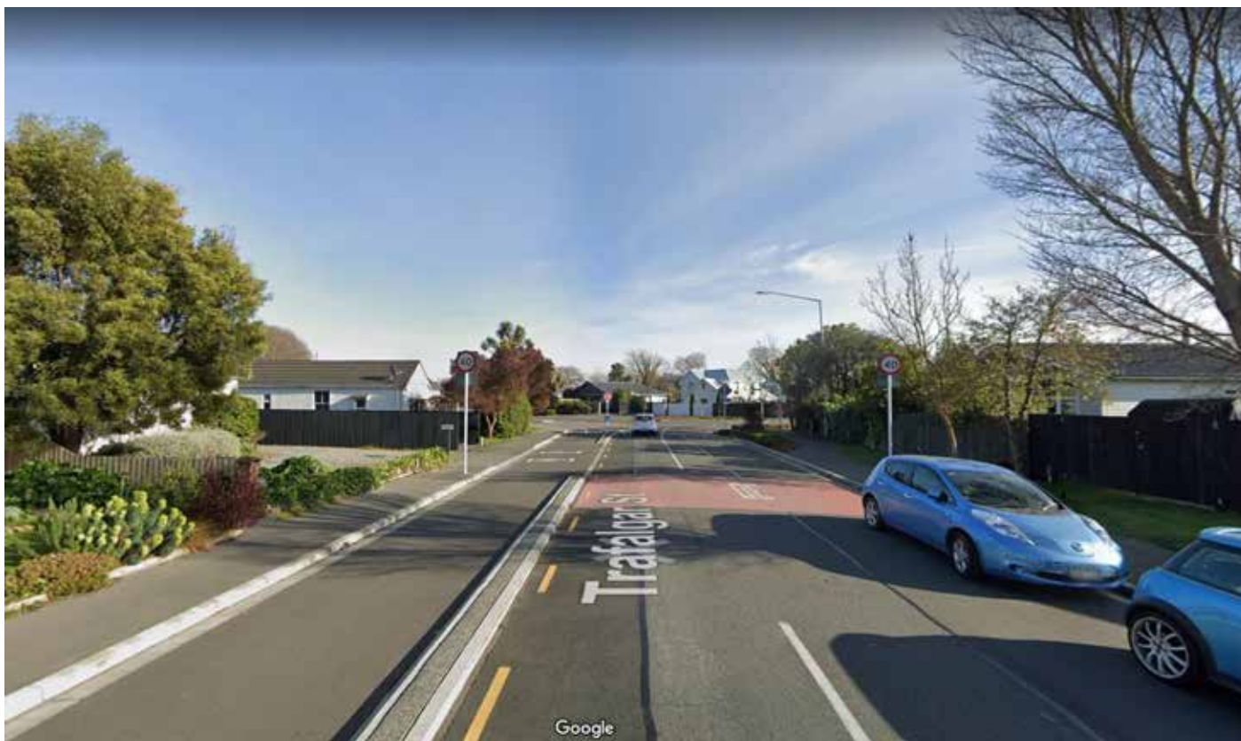
Concrete kerb separator - bi-directional cycleway:
