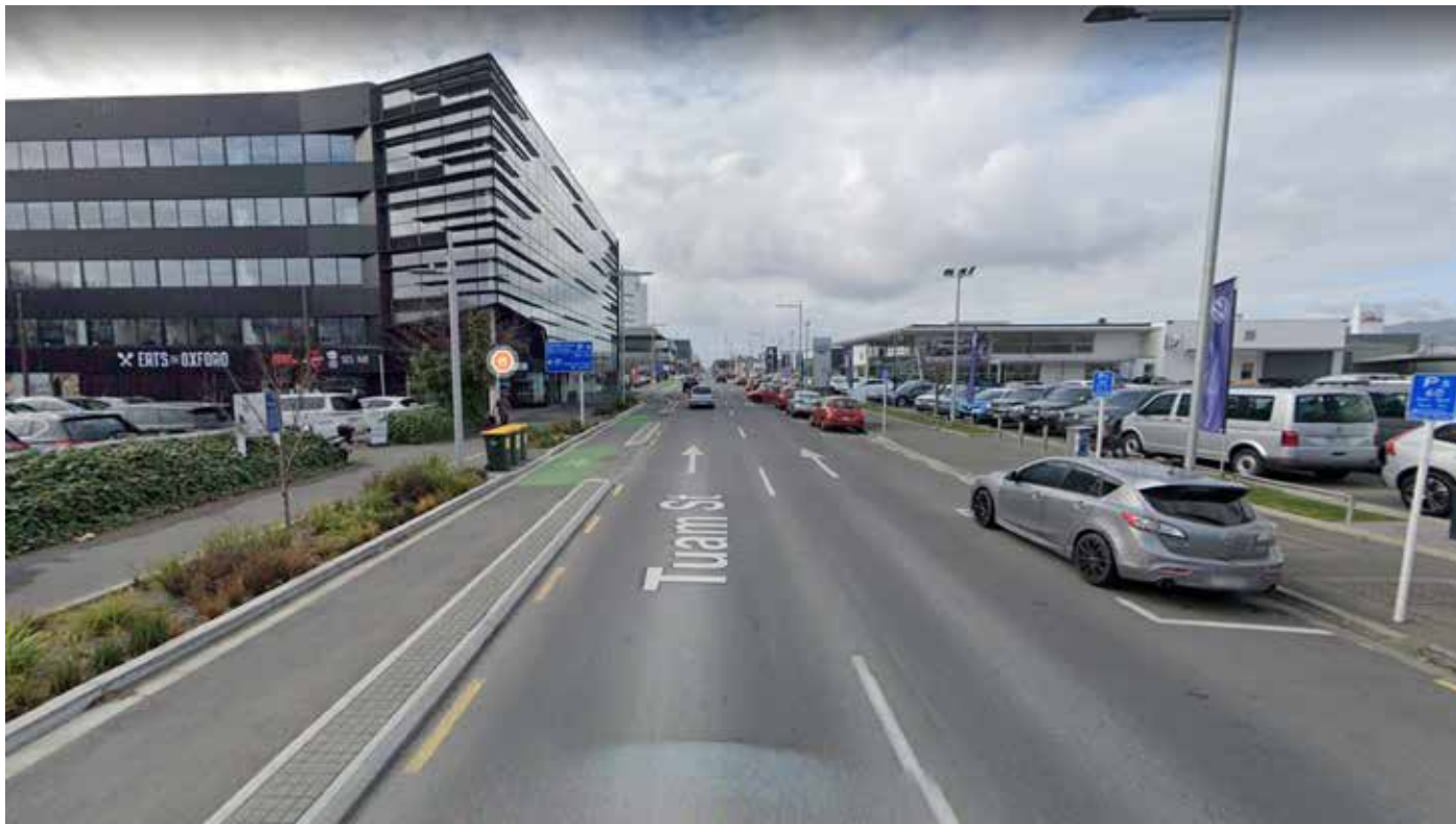
Concrete kerb separator - bi-directional cycleway:
