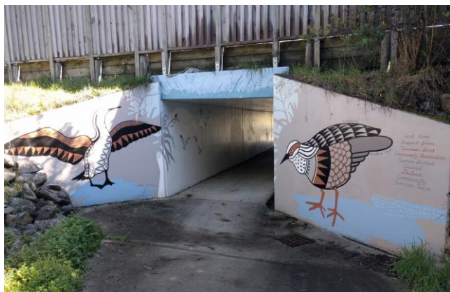
Highway underpass just east of the walkway.
