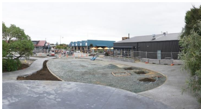
Hard landscaping underway, June 2021
