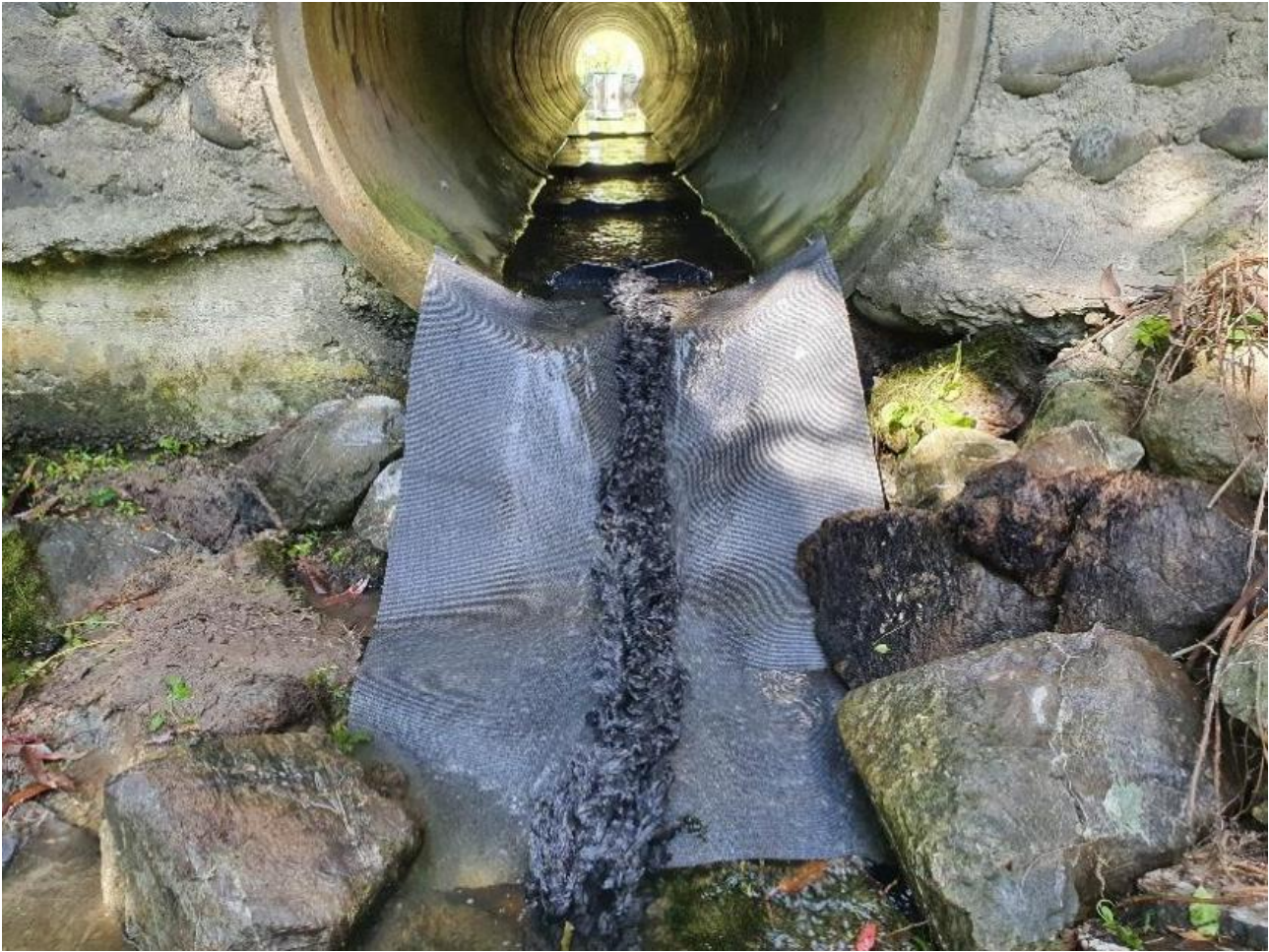
Figure 2. Example of a flexible ramp and mussel spat rope combination to remediate a perched culvert (Williams Creek).
