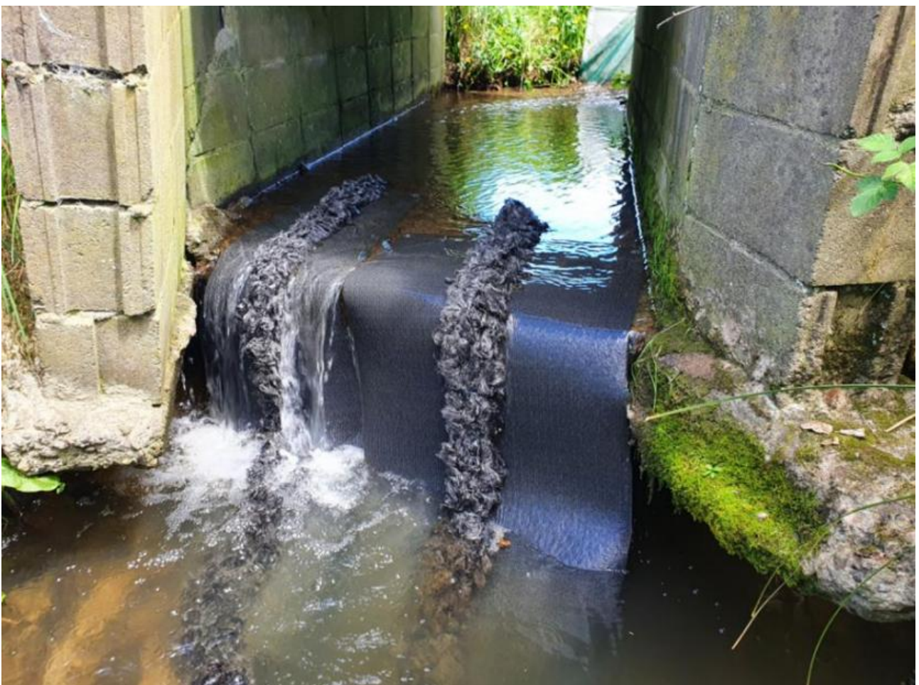
Figure 3. Flexible ramps with mussel spat ropes installed at Harley Creek culvert.
