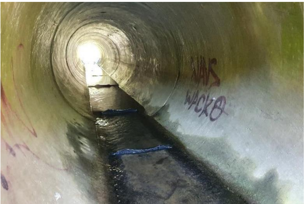
Figure 1. Flexible 'weir baffles' installed inside a pipe culvert (Williams Creek).
