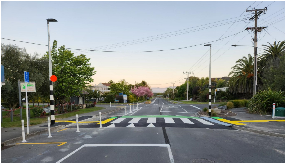
Figure 3 Raised Pedestrian Crossing Close to Higgs Road.
